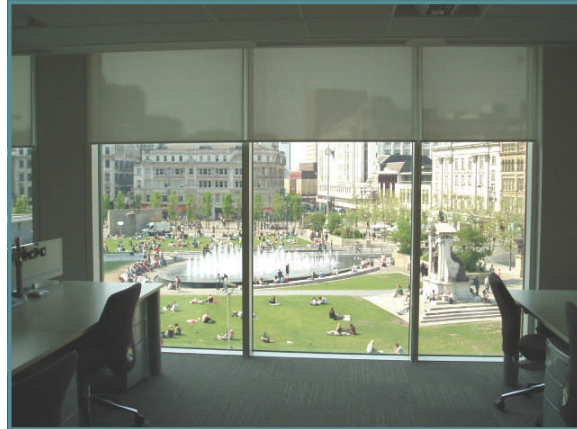
Blinds partially deployed
