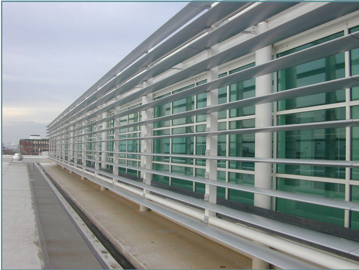
Brise Soleil to first floor windows
