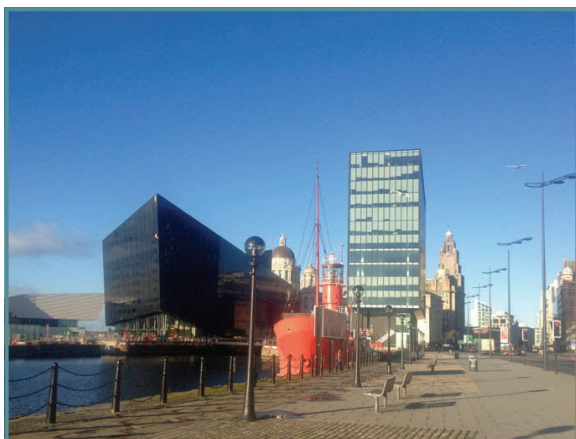
13 storey office block
