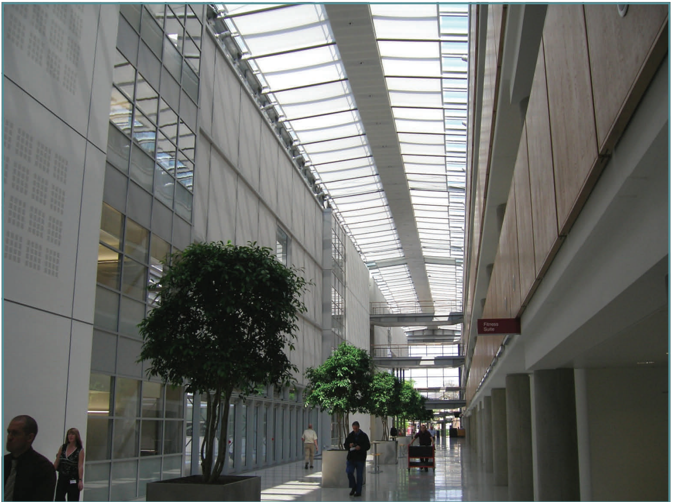
Main street atria blinds partially deployed
