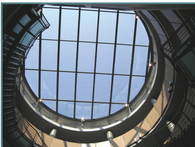
Drum atrium blinds fully retracted
