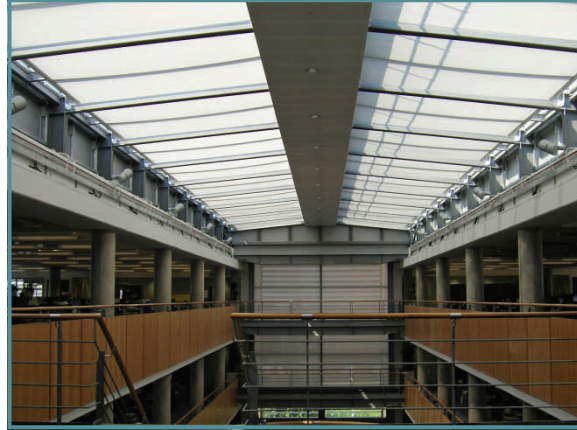
Wing atria blinds fully deployed
