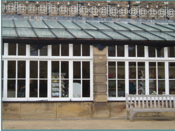
External view showing old glazing
